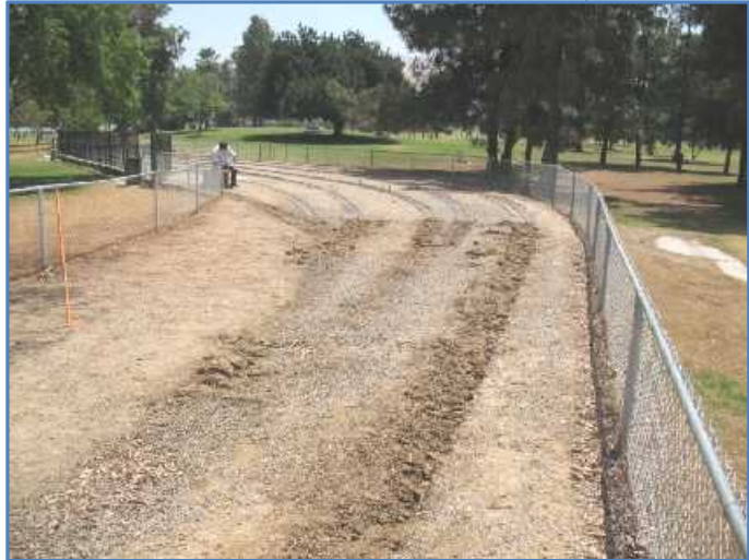
More track was removed... that translates to more work-day “fun” at the RLS!
