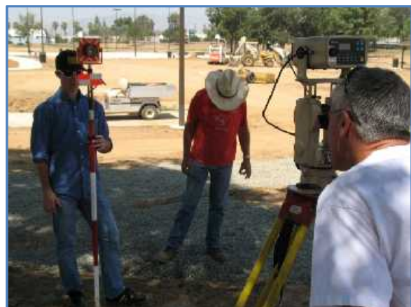
The Bunts’ Survey Team (Dave, Don and Tommy) get laser accurate readings of the north lead into the new Iowa Yard and Station.
